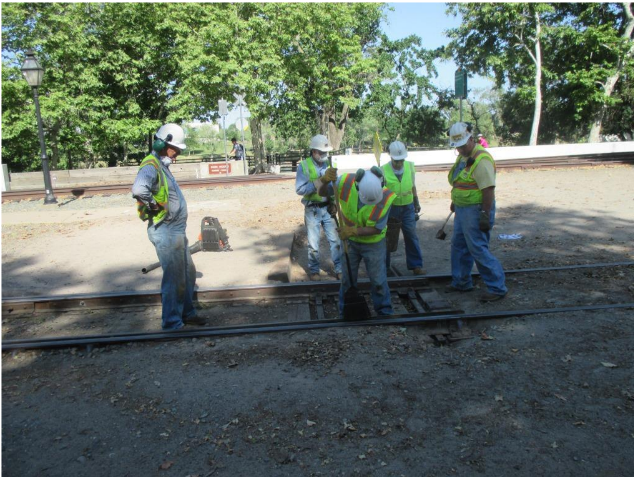
Mike W. removes debris from between the points and stock-rail
